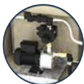
Pump pre-installed with rain/mains changeover
