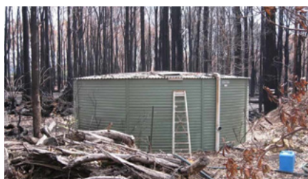
Figure 1: Steel water tank unaffected by bushfire
