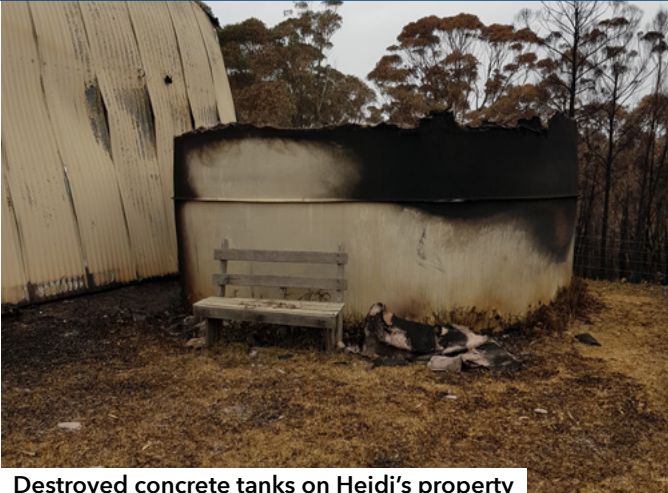
Destroyed concrete tanks on Heidi's property
